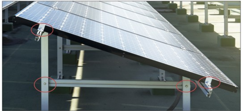
Examples of PV Racking System Fasteners
